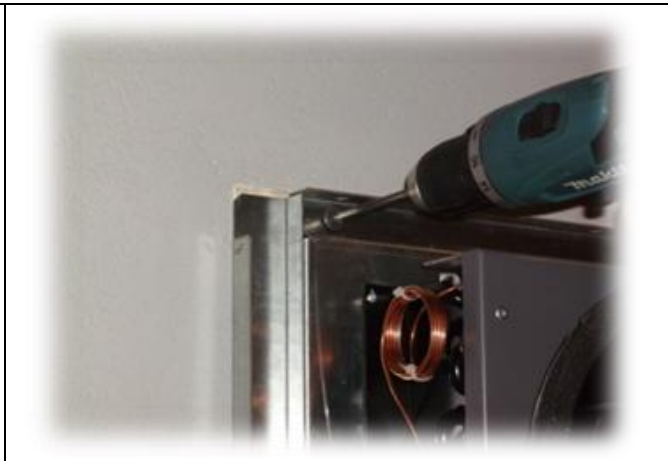
Tighten the two screw/washer units at the top
