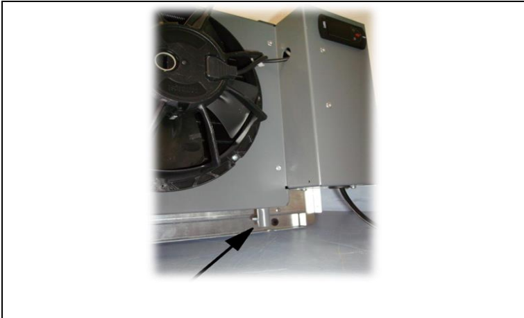
Flow from the condensate collection tray.
