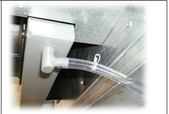
Push the PVC pipe on.
