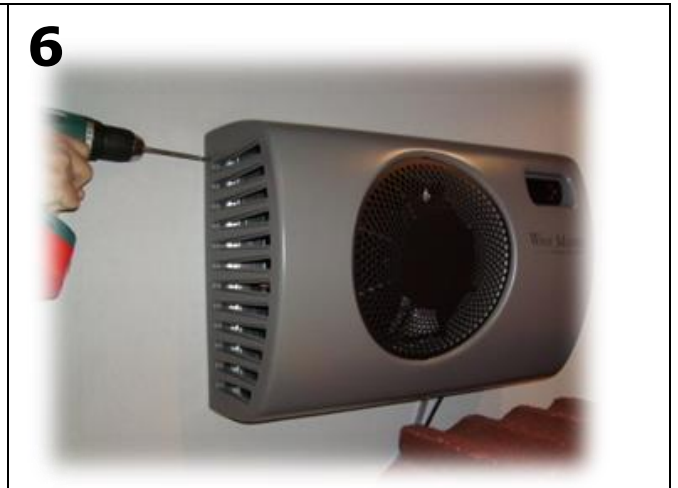
Refit the cover on the Winemaster and tighten the 4 screws
